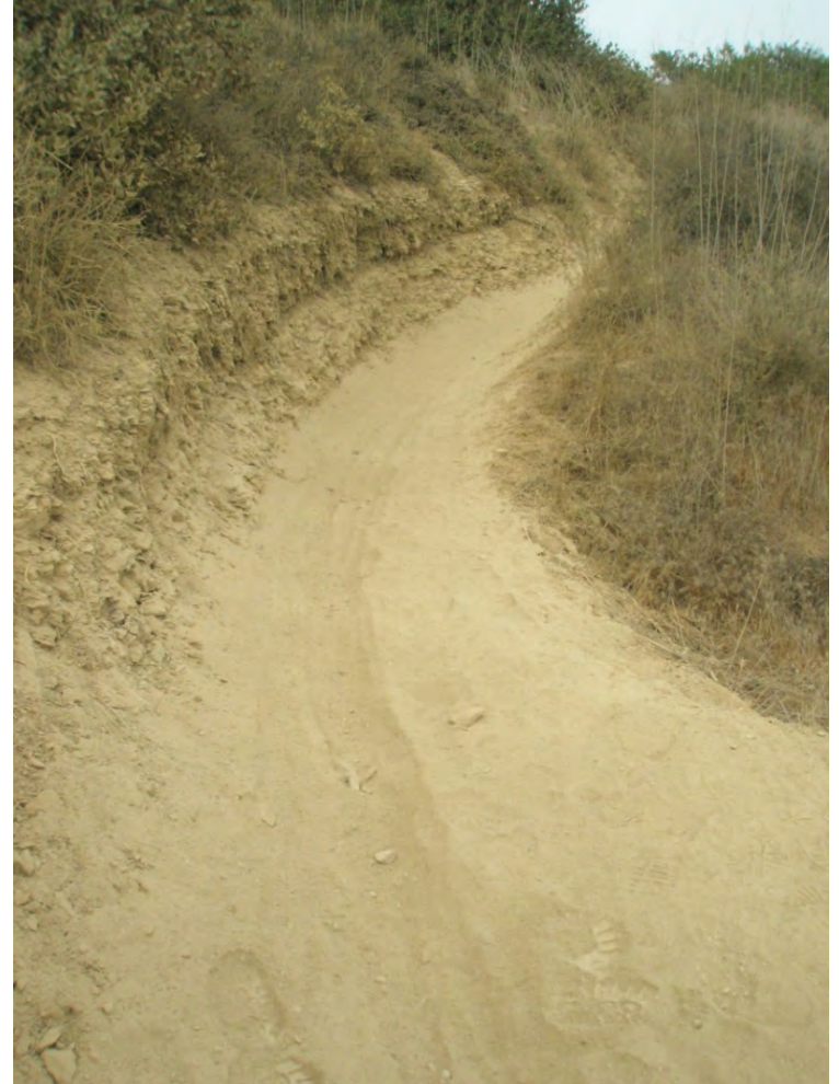
The above photo demonstrates the trenching that can occur when a trail characterized by dry, powdery soil sees considerable use by mountain bikers. July 2009
